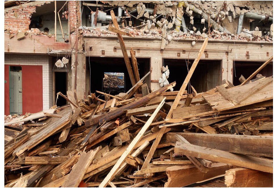
Construction timber from urban mining, one type of wood waste
